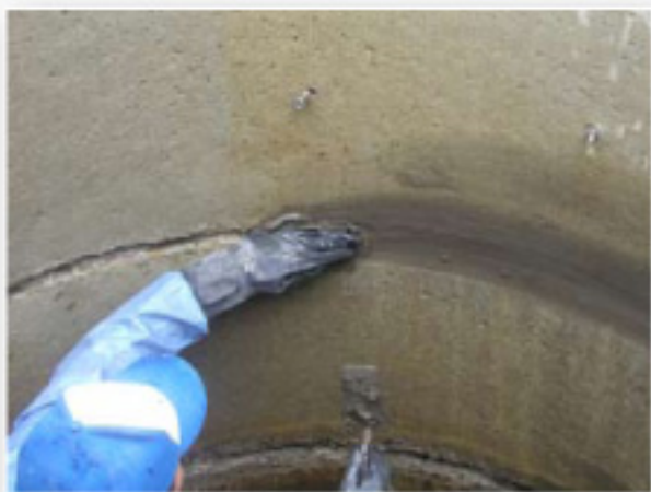
Sealing leaking joints
