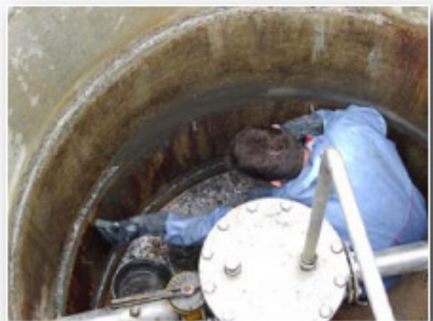
Sealing of leaking points
