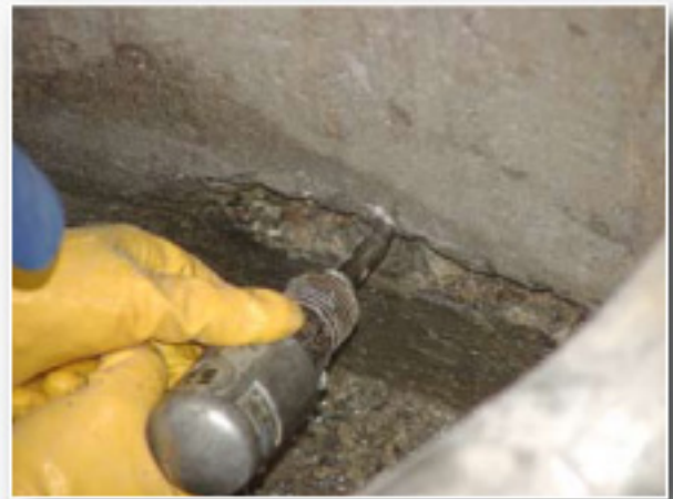
Substrate preparation
