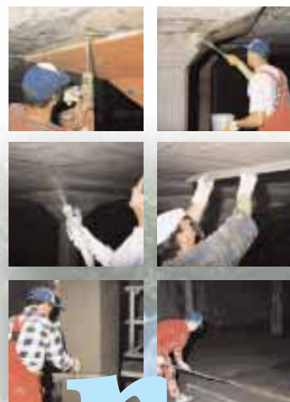
VANDEX CEMLINE MORTAR and VANDEX CEMLINE TOP GREY. Application mechanically and by hand.
