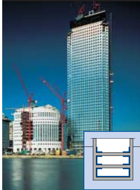
Structural and industrial engineering
