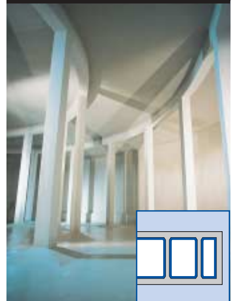
Drinking water reservoirs
