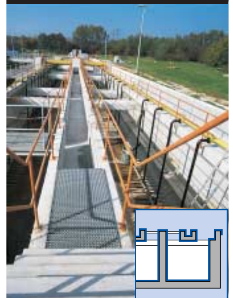
Sewage treatment plant
