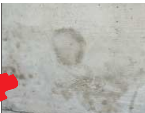
The water leak is stopped permanently.
