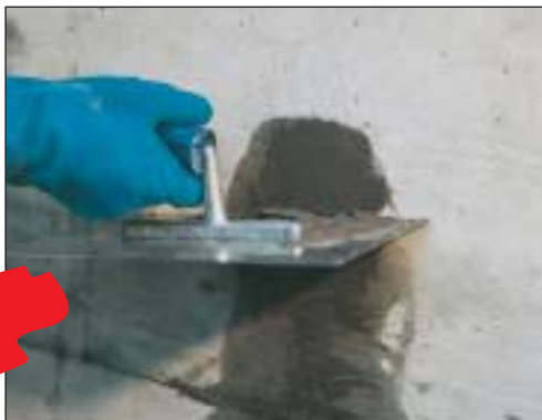
Level off surface.
