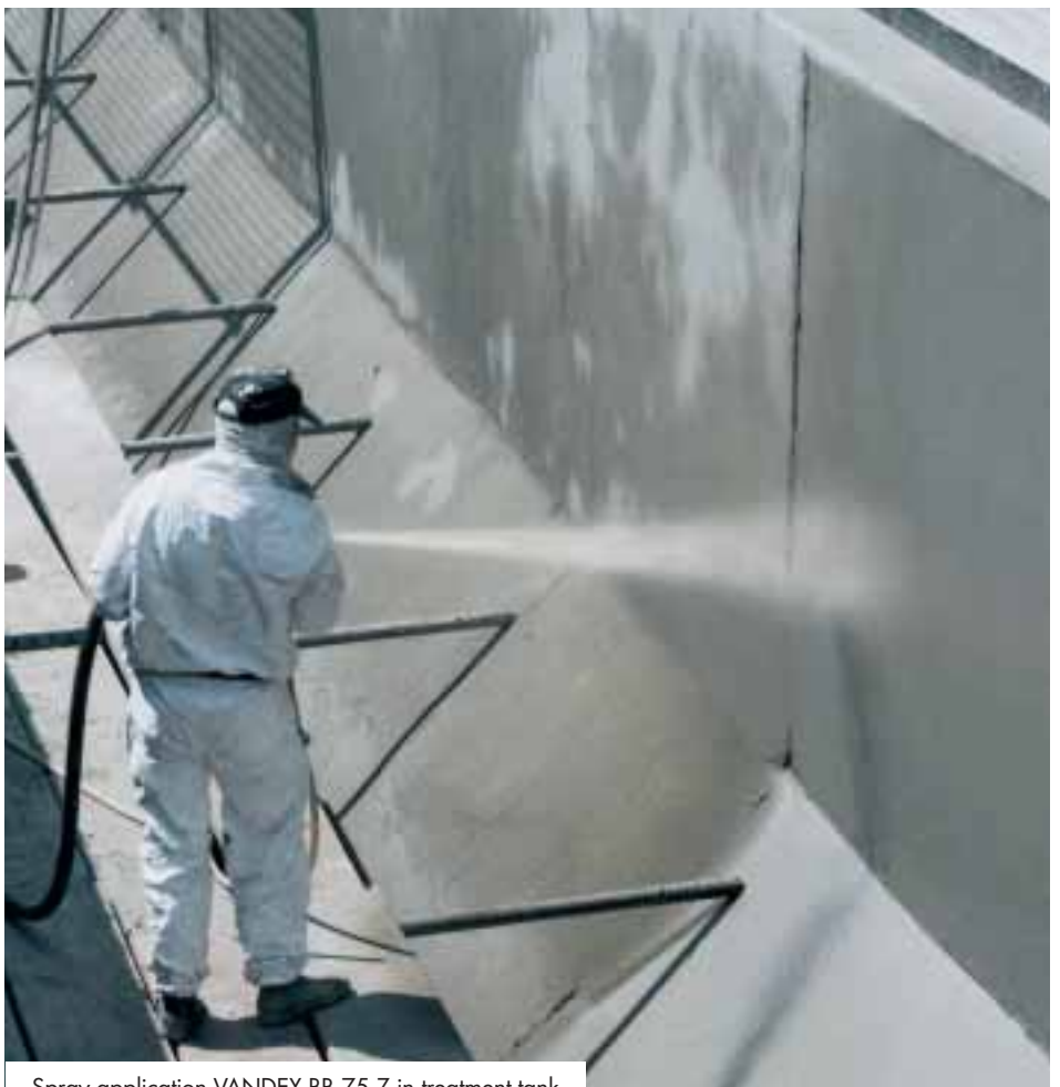
Spray application VANDEX BB 75 Z in treatment tank
