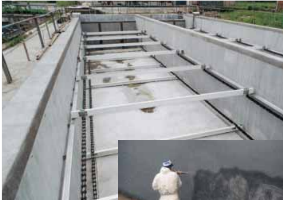
Spray application VANDEX POLYZEM Z
